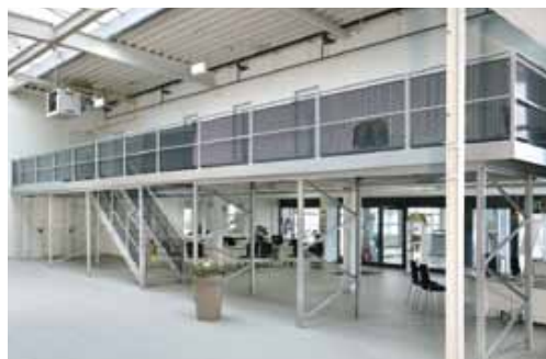
This META steel platform provides space for employees in 8 office rooms
