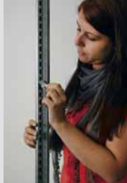
Step 2: Attach shelf clips
